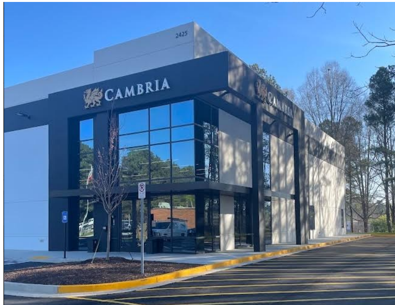
The new Cambria Sales and Distribution Center in Duluth, GA. Photo credit: Cambria
